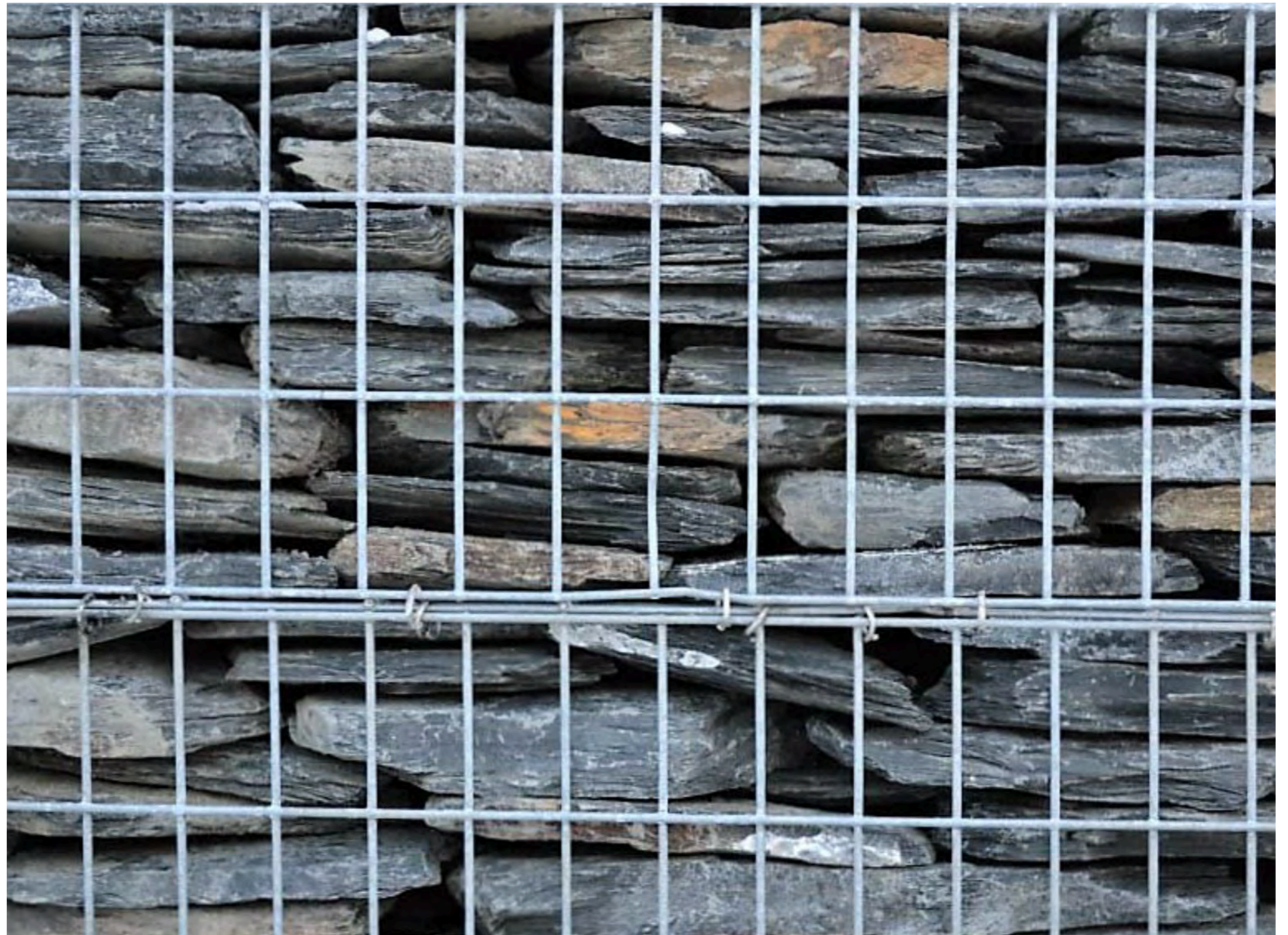
Slate in a gabion basket can contribute to the overall aesthetic while create voids for habitat
