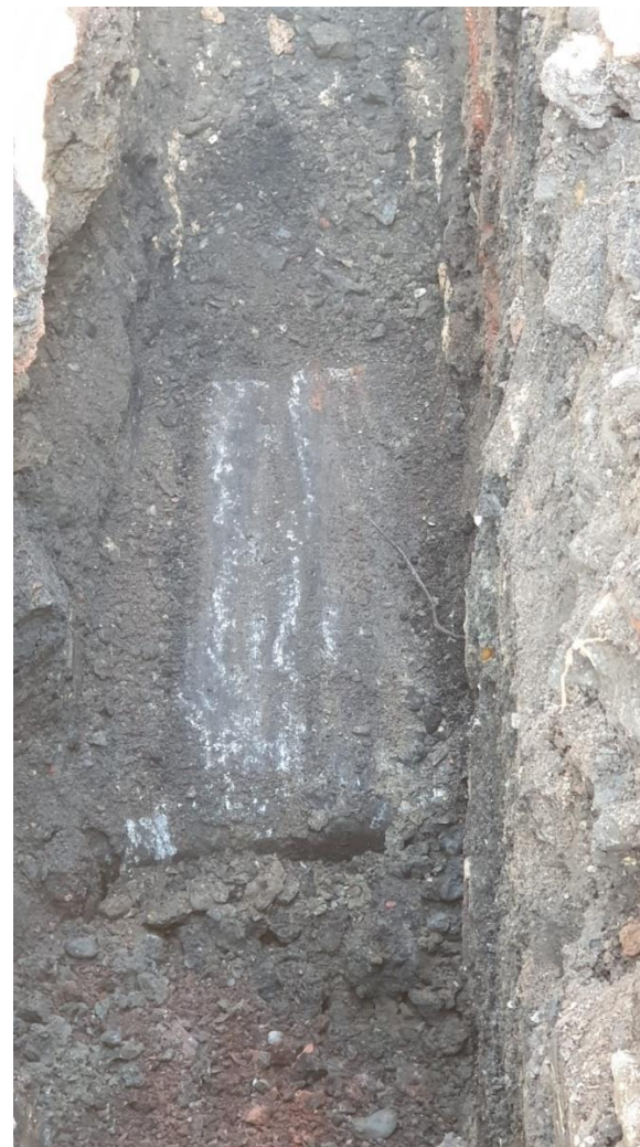
Plate 2: TT101 from west showing suspected former dock wall
