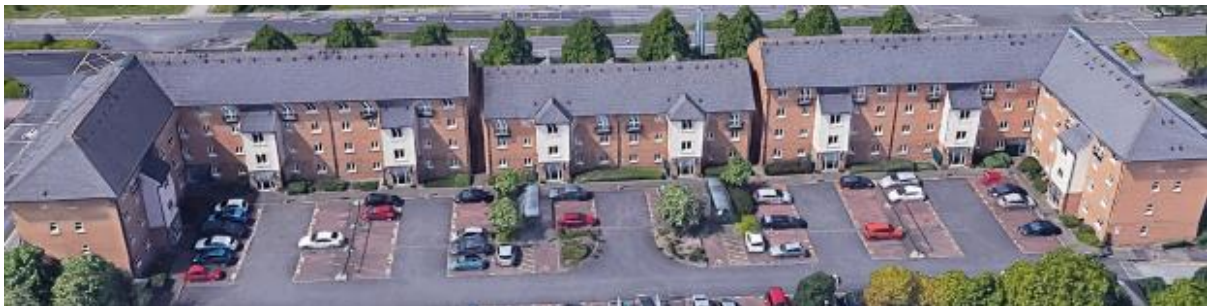
Figure 20.1 View of façade assessed for Existing Residential Building E2 on Llyod George Avenue.
